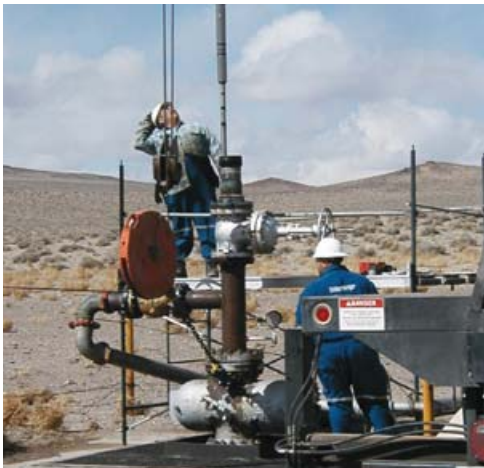
Drilling exploration crew performing initial well logging tests at the Desert Peak site, Nev. PHOTO: DOE/NREL, Pat Laney
