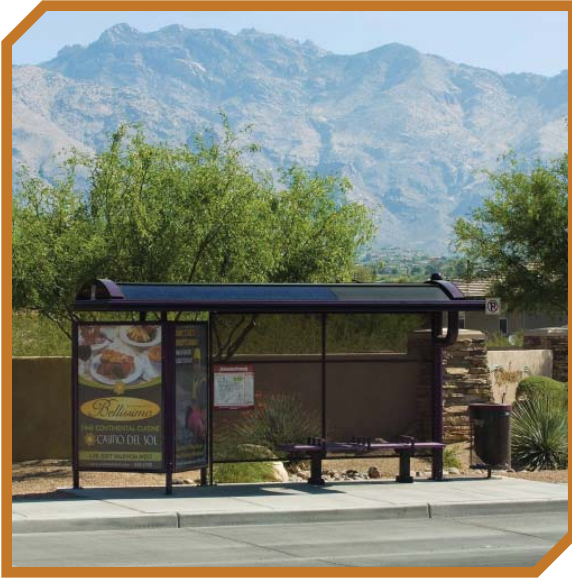
PV on bus stop shelter.
