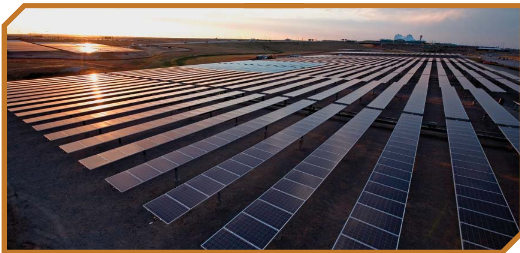
Denver International Airport, with a commitment to energy efficiency, has built the largest solar farm at a commercial airport in the United States. Photo courtesy of D.I.A.
