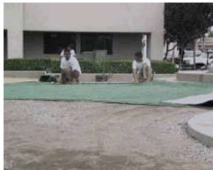
Synthetic Turf Rolled Out After Removal of Turfgrass
