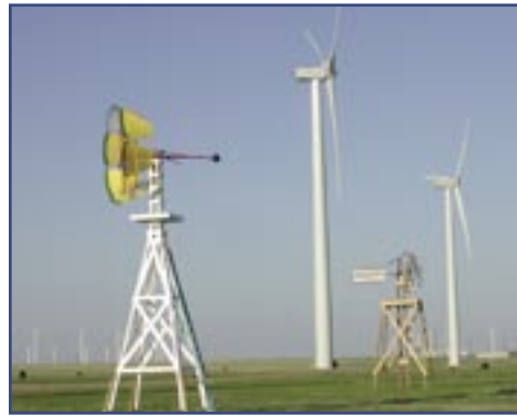
The past meets the future of wind energy at the Colorado Green Wind Power Project.
