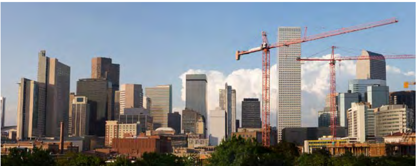
Construction in Denver, CO.
